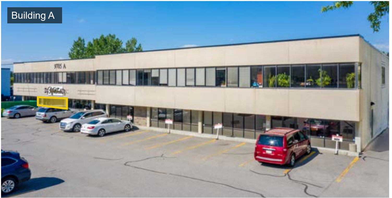
Building A | Back
